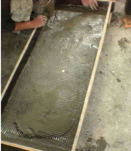
Fig 2: Placing the wiremesh
