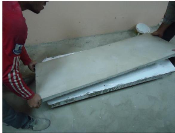
Fig.5: Placing the ferrocement cover connected to repaired slabs by epoxy
