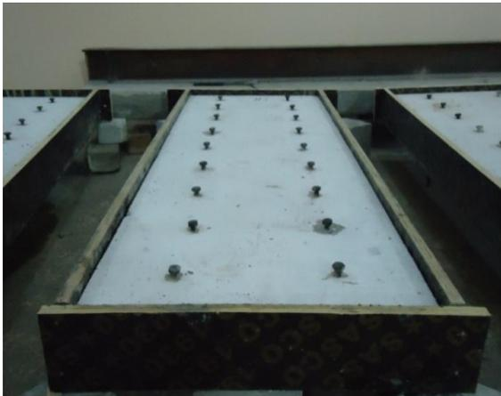
Fig.4: Placing the bolts to connect the ferrocement cover and repaired slabs
