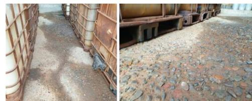
Fig.1 Sulfuric acid impact on warehouse floor in Mosul industrial area.
