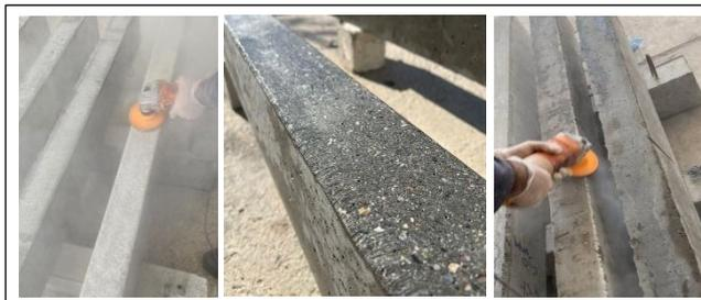
Figure 6: Surface preparation prior to CFRP application.
