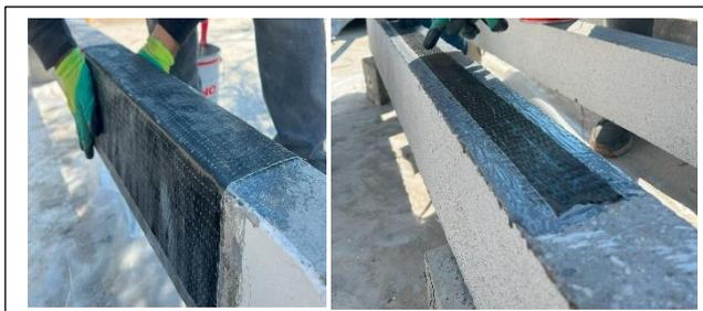
Figure 7: CFRP application.
